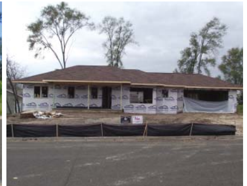
New Construction in Progress at 907 8th Avenue
